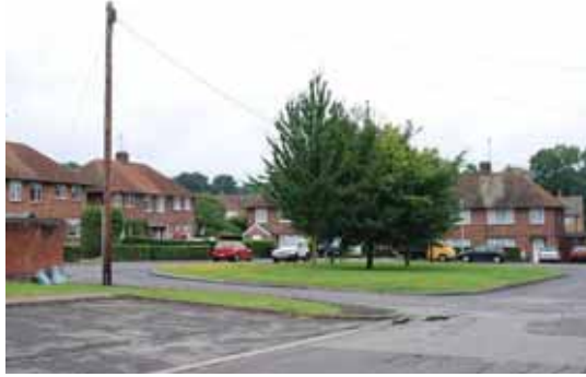
Houses arranged around areas of shared amenity greenspace, as in this example from Windsor.
