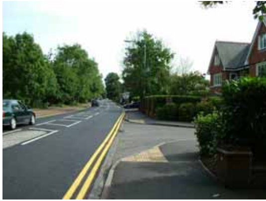
Street proportions are relatively wide with properties set well back from the main road (Maidenhead Riverside).
