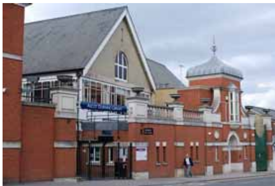
Architectural detailing contributes to visual interest, as seen here at Ascot.
