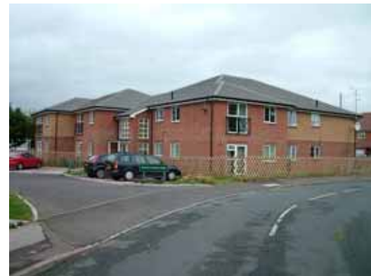
Area 11I Trenchard Road, Maidenhead
