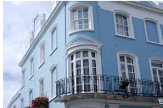
Regency style buildings have greater decoration, including distinctive moulded stucco (Windsor).
