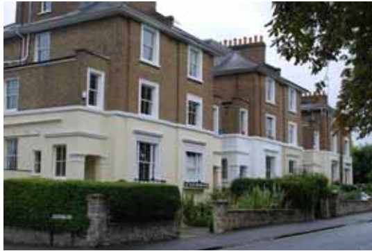
Buildings often have grand proportions, as seen in this example from Windsor.
