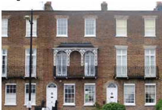
Plain, elegant brick façades with decorative wrought iron verandas and fan lights, as in this example from Windsor.
