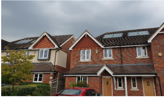
Climate concerns have prompted measures like integrated solar panels in new builds
