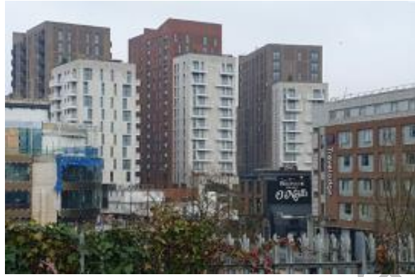
Recent high-rise blocks in the town centre have been widely criticised for their height
